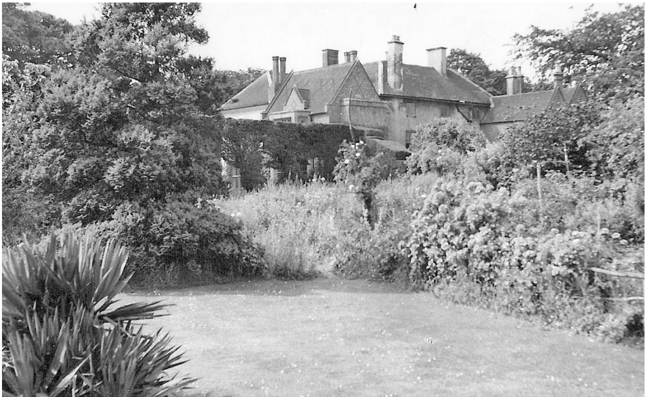
This picture taken from the north east shows how extensive the rectory was behind the frontage shown in the top picture. The nearest part of the building with the mock Tudor chimneys is in the style of the Church House and is thought to have been built by the Rev. Robert Miles in the mid 18th C.
