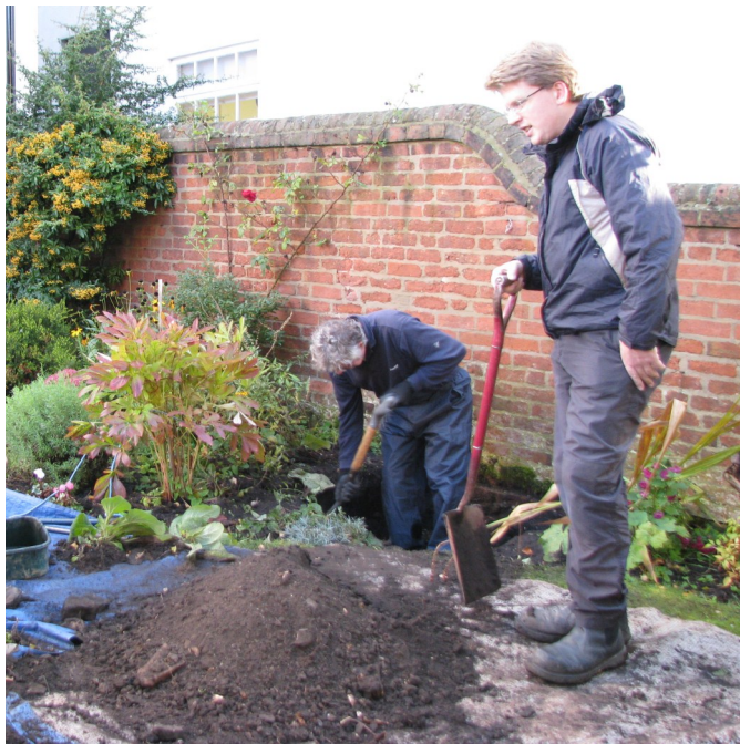
Digging pit CB01E
