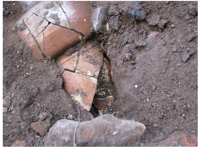
Close up of the junction in the drain. It was broken before the pit was dug and flows towards the house.
