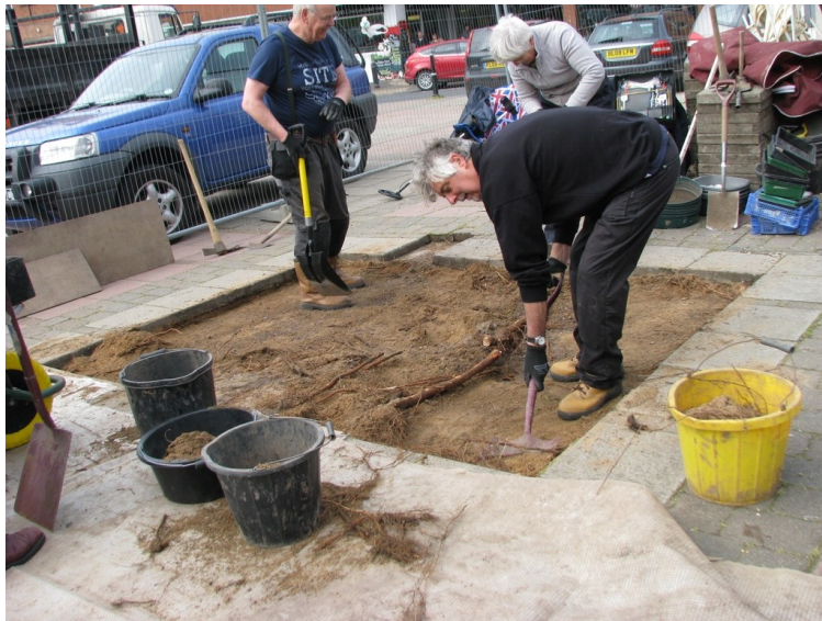
Starting work on the excavation. The flags have been removed and the underlying sand layer is being taken off.
