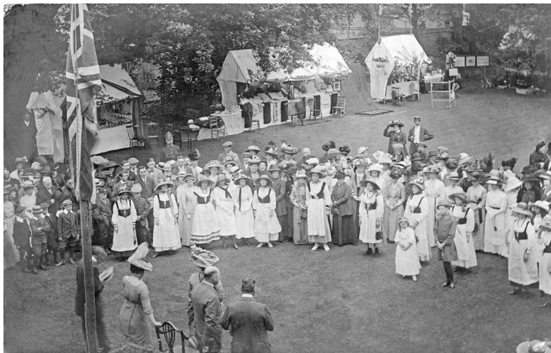
Fig 17 Flagpole in the front lawn of the garden. The clay wall between the school grounds and No 7 Church Street is behind the tents at the top of the picture.
