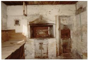
So-called 'patent' ovens were introduced later in the 19th century, in the main developing cleaner and better controlled ways to heat the oven. These were more costly to build and the side-flue oven was not adaptable. The latter was still the most common type in use in 1900 (Vine). A similar type of oven to that in Bingham now on display in Mill Green Museum in Hatfield, Hertfordshire, was used between
