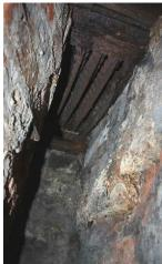
The interior of the oven proved awkward to measure. Measurements that were made from the oven entrance indicate a near but not precise circular shape, about 10¾ feet (3.27m) in diameter. In profile it consists of vertically set bricks at the side and then
