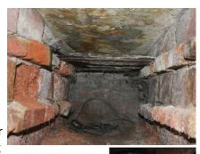
to conserve heat (right). (BHTA note: if the oven interior **is** from the 18<sup>th</sup> century, might this have been the furnace area, commonly introduced when the practice of burning kindling inside the oven was superseded, to prevent damage to the oven tiled floor, and before the introduction of the side flue?)
