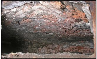
a gradually curving domed roof which at the centre is 18 inches (45cm) high. This shallowness would have helped to radiate heat back onto loaves to create a light spongy top (Hardyment 1992, 112). The oven base is now covered in debris but it probably has a covering of tiles and some of these may have been re-set beneath the oven frontage during.
