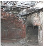
To the right of the oven some blackened firebricks that project into the oven can be seen (left), along with blackened bricks in the oven's roof.
