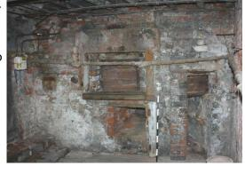
appears to have replaced an earlier stone as part of the latter survives to the far right beneath the stone jamb.
