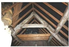
The two trusses are simple A-frames with high collars, all built from insubstantial timbers that although almost certainly original to the house had too few rings for dating purposes (left). The parts are pegged together; no assembly marks were seen. In contrast, the attic space in the east part of the building is completely modern and set off a higher floor level (arrowed, right).
