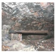
To the left of the oven door there is a small former opening where air for a draught to control the heat entered the oven; this is now blocked by three bricks. Closer to the left stone jamb a circular metal tube has been inserted through the brickwork for a pipe to enter the oven (left). This is possibly a replacement device for controlling or even heating the air within the oven; this may warrant further investigation.
