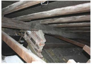
The roof has clearly been altered and part of the evidence are two redundant long beams with mortices showing that now run along the centre of the attic floor (arrowed, right).
