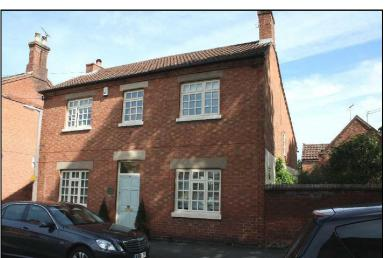
this was not evident. It is principally brick -built but has stone dressings around the openings. All the brickwork at the back is painted white and parts of the side walling are painted or rendered over. The roof is covered with modern pantiles and slopes back from a ridge over the axis of the south
