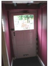
The front door (left) has fielded panels (a raised or recessed panel) with a wide flat surface surrounded by moldings with a shallow one to base, suggesting that the door may have been turned through 180 degrees and the lower panel removed to take a window.
