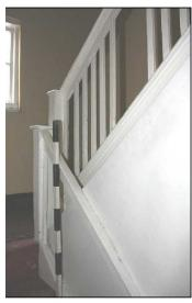
The rear stair-turret contains a dog-leg staircase with a lit rear landing between each floor. Each rise has 5 steps. The staircase ( left) itself is of simple design and almost
