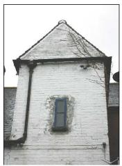
added cell with the catslide roof to its left of the turret and a lower addition, set-back to its right. Whilst the street walling is one brick thick, the side and back walling is thinner and floor joists can be seen exposed at the back.
