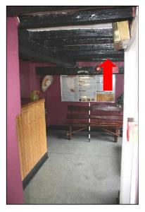
The central wall has been largely removed at ground and first floor level, being replaced by a central (red painted) brick pier and boxed-in timber or metal beams above where the wall had been (below, right, red arrow)).
