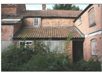
Part A4/B4: A part single -storey, part two-storey lean-to addition was made at the rear of Parts A and B at some point in the mid-20th century. The two-storey section incorporated a corridor and a small room on each floor, whilst the single-storey section, with its thicker walling, contained a new kitchen.
