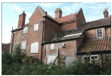
The brickwork on the side and rear elevations is different with headers and stretchers laid in irregular coursing, the bricks being about 2¼ inches (57mm) thick and 9¼ ins (235mm) in length. The east side, the stair turret and the central stack feature a dentilation course. The gable ends of the main range and the
