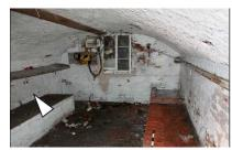
The cellar (left) is sizeable with its walls just stepped in from those above ground level by a matter of inches, giving dimensions of about  $3m \times 5m$  ( $10ft \times 16\%ft$ ). It has a barrel-shaped roof and low thralls on either side. It was lit by a now blocked up sunken light in the west wall . A straight joint in the east wall suggests that there may have been a recess under the stairs and that the thralls may have been added later.
