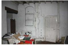
Rooms 1 and 2 at ground floor level were originally accessed through a near-central lobby next to the stack which one entered through a doorway from the stair turret. This doorway has been blocked off and new doorways created in the east wall of both rooms . The lobby provided direct access into Room 1, whilst another
