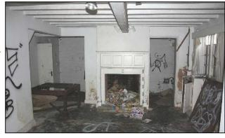
brickwork showing in the back wall (not covered by plaster as elsewhere) and evidence of a brick floor surface 25cm down made of bricks 2½-2½ inches (57-63mm) thick, suggestive of a late 18th century date. On the upper floor there is a single bedroom (Room 15) with a fireplace (left).
